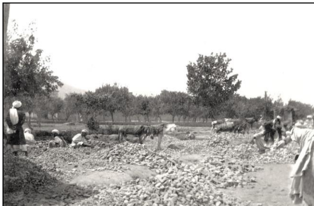
Strassenbau / Road construction in Kandahar
